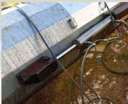
Slip on joint by hydraulic jacking system
