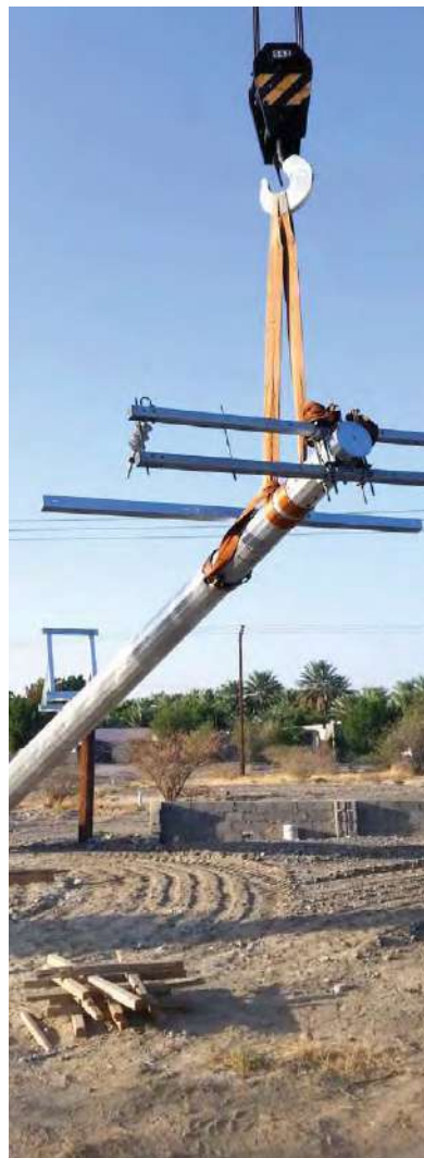
3 SLINGING AND ERECTION
