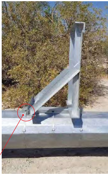
CABLE SUPPORT (SINGLE BAND-IT TO BE USED)
