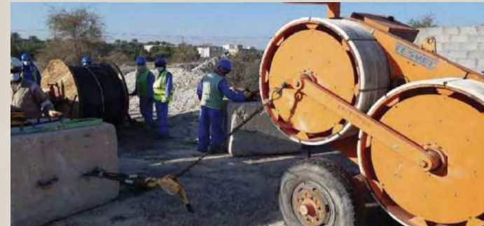
TESMEC (tensioner) Model. 611/675/10 Max tension 75 kN
