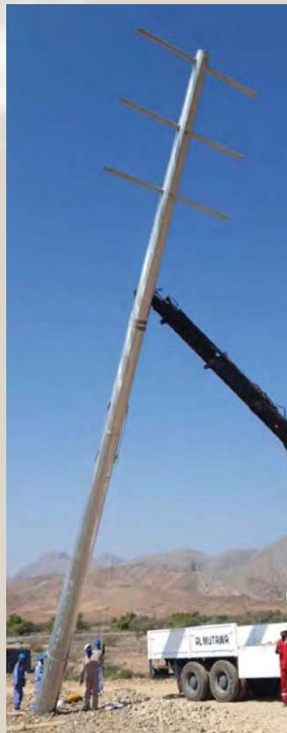
3 SLINGING AND ERECTION
