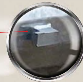
SEMI-BOLLARD WELDED ON POLE TO PERFORM THE SLIP ON JOINT
