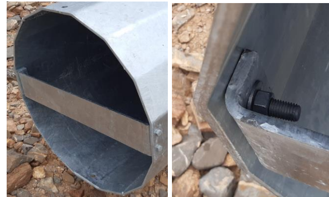
Method for danger plate installation on steel poles
