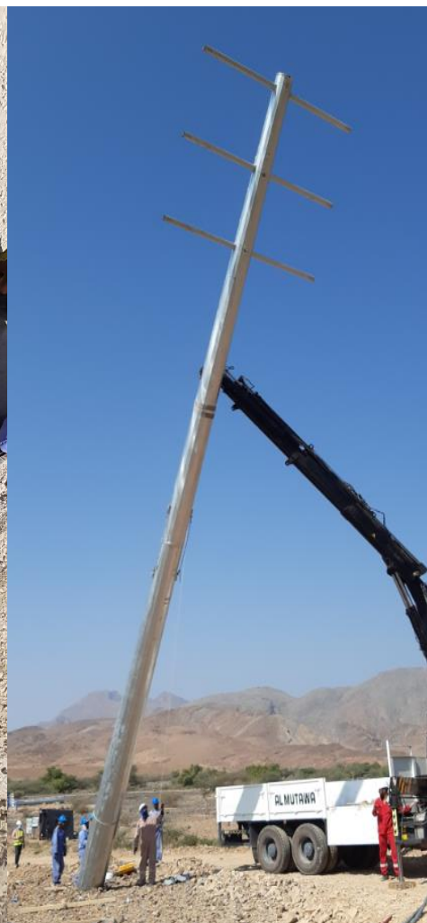
3. Slings and erection
