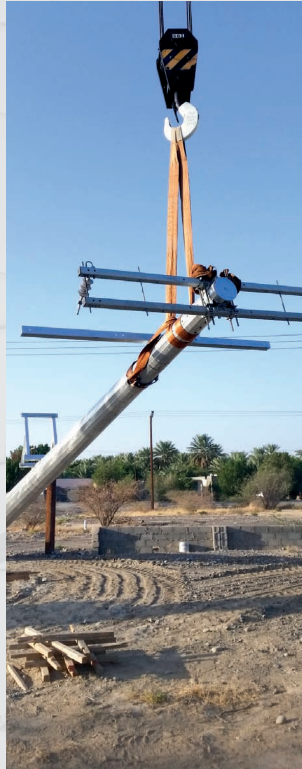
3 SLINGING AND ERECTION
