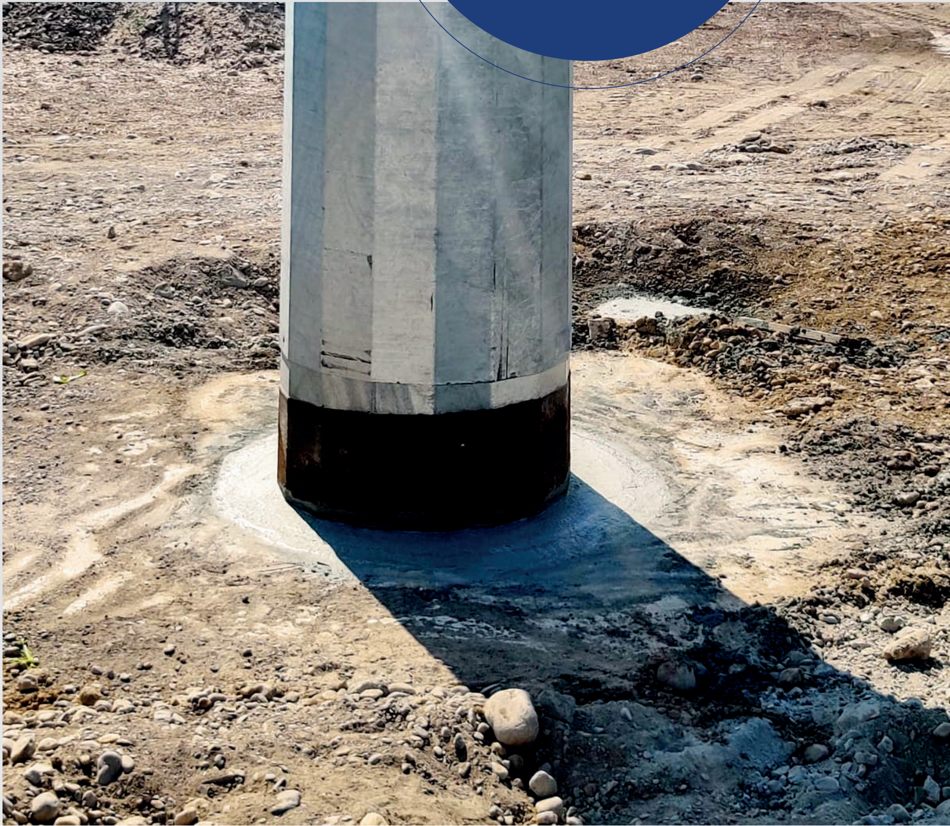
BACK FILLING ON CONCRETE
