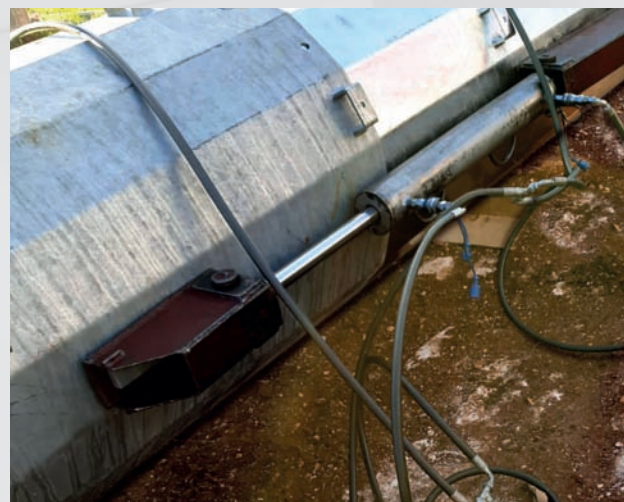
Slip on joint by hydraulic jack
