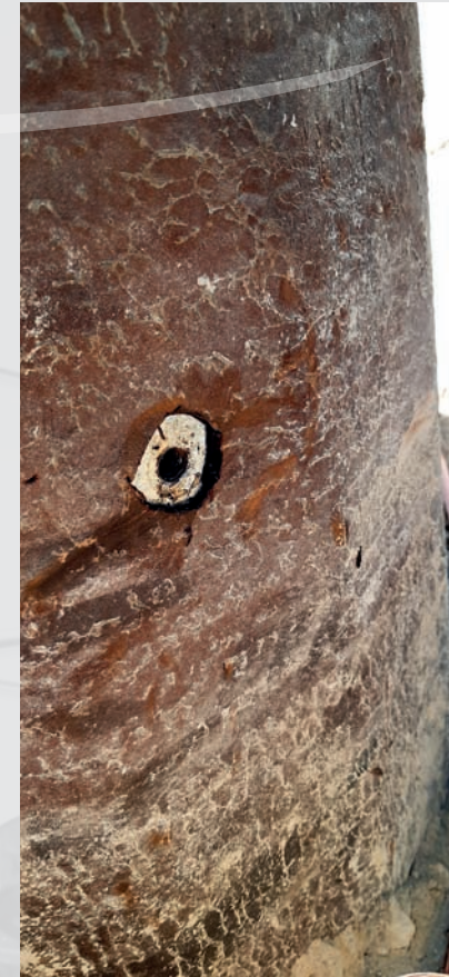
Earthing plugin stallation the pole
