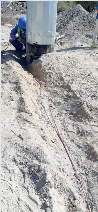
Copper cable installation
