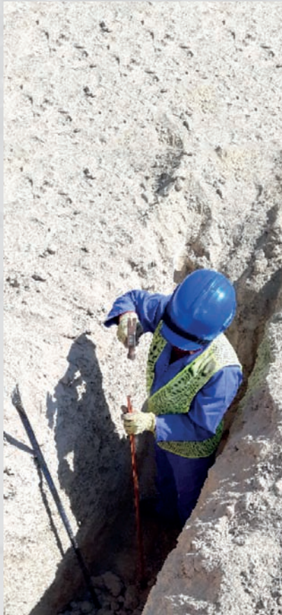
Excavation and copper bar installation
