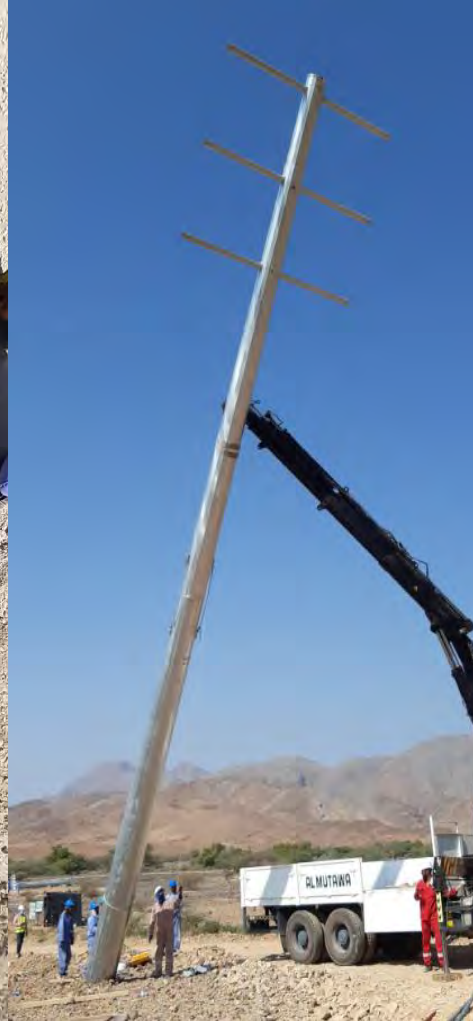
3. Slings and erection
